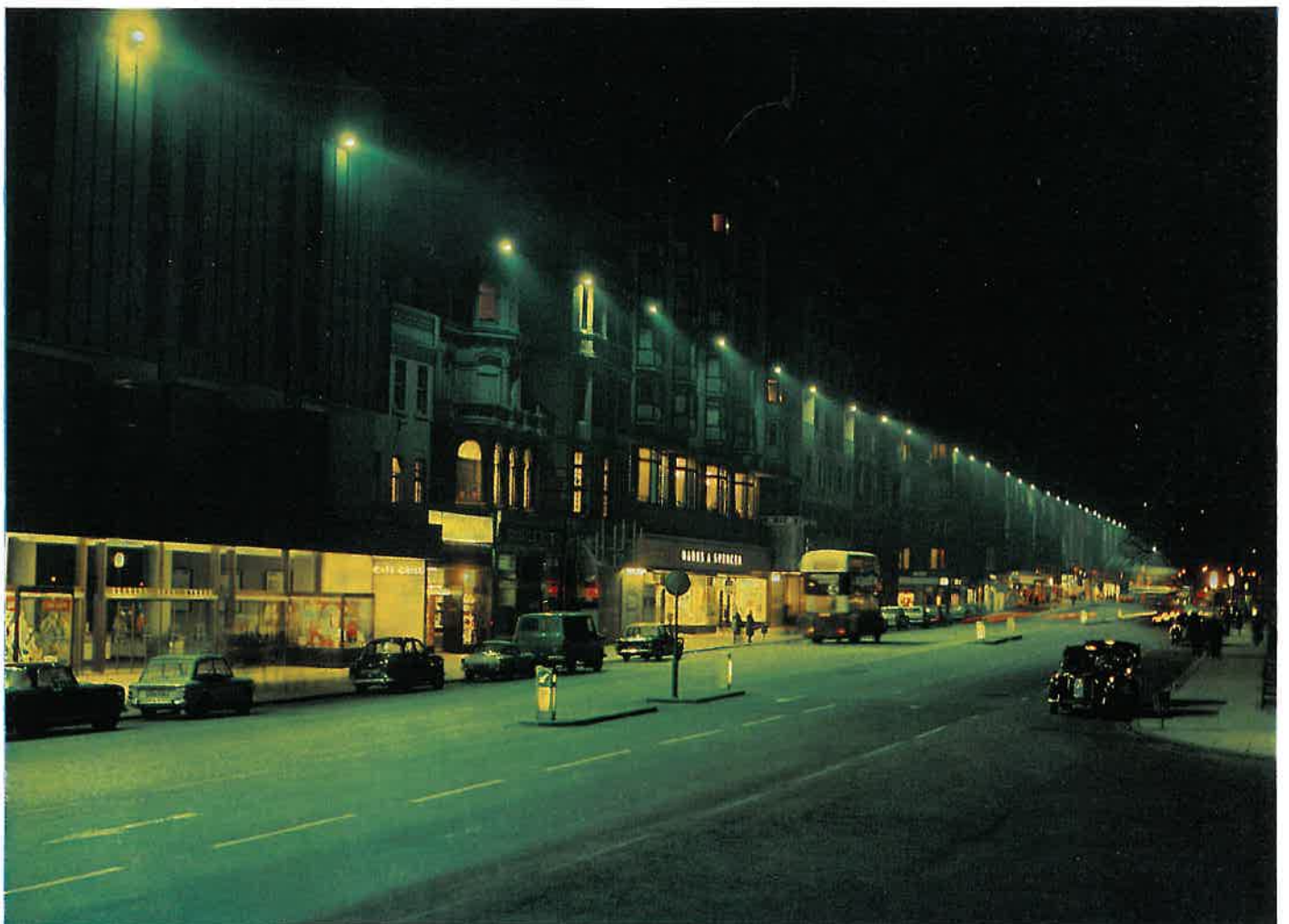
Below Princes Street, Edinburgh, lit by Mazda linear mercury halide lamps.
